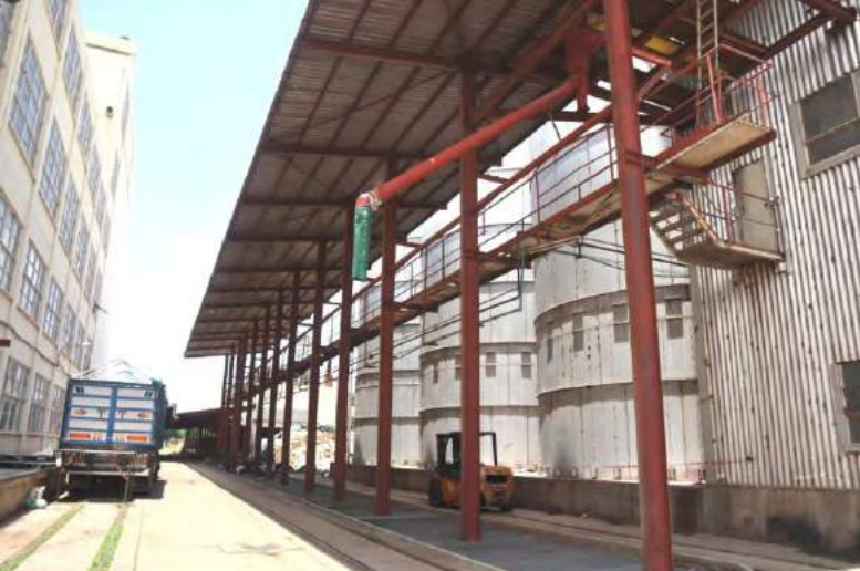
Raw material intake
